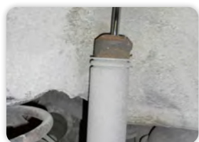
Loose bump stop
