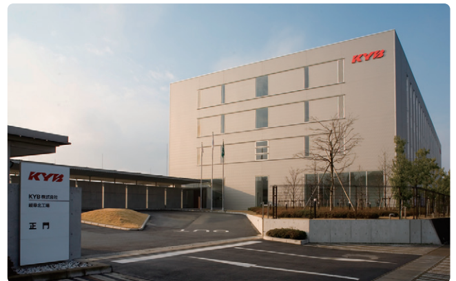
Gifu North Plant
